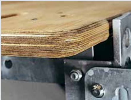
45 mm thick platform decking made of bonded multilayered plywood boarding.
