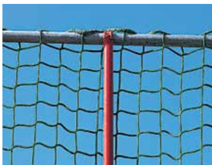
The safety net is simply threaded onto a scaffold tube.
