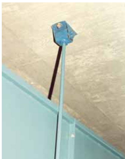
Belt conveyor hanging on type V
