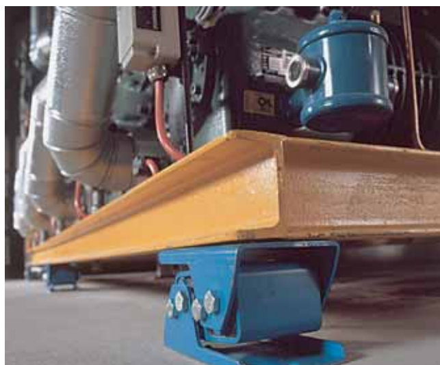
Cooling compressors on type ESL mounts
